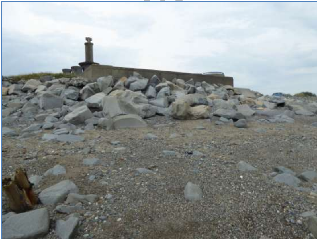
Plate 4: Protection to Dwr Cymru Holding Tank
