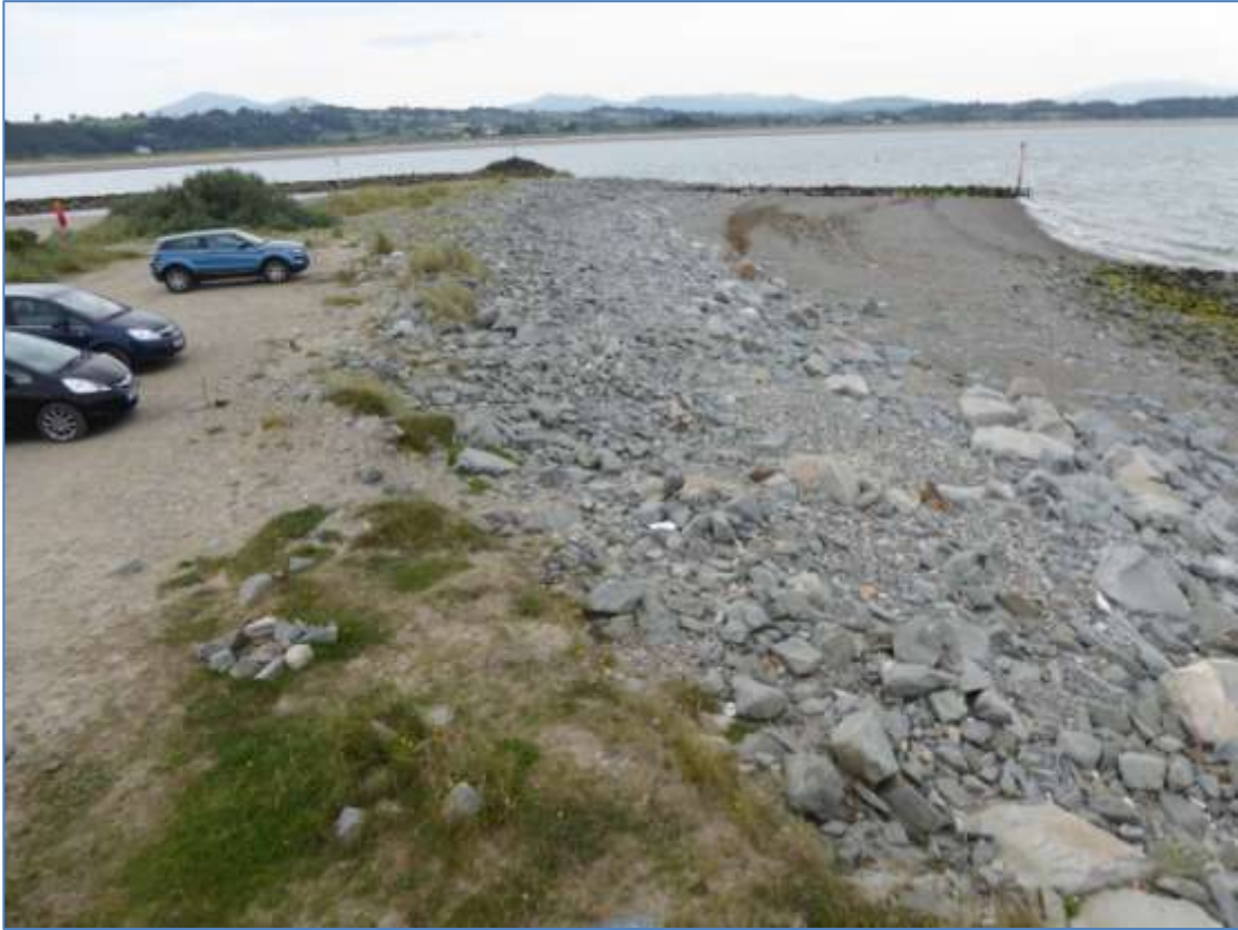
Plate 5: Foreshore between Dwr Cymru Holding Tank and Crib Groyne
