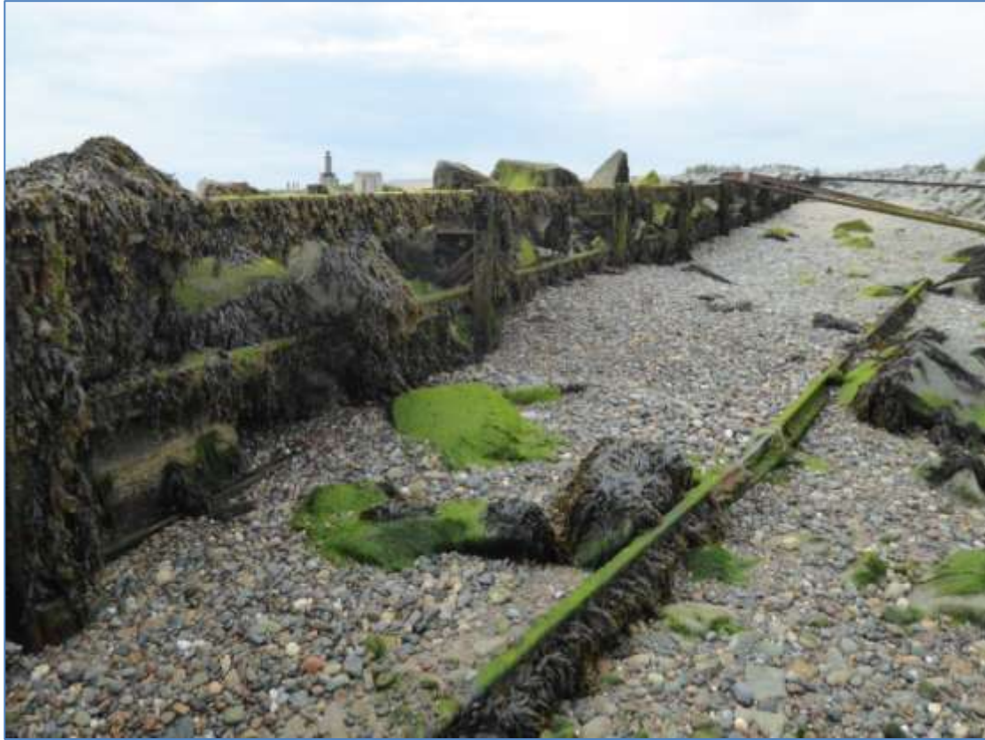
Plate 11: Elevation of Crib Groyne on downdrift side
