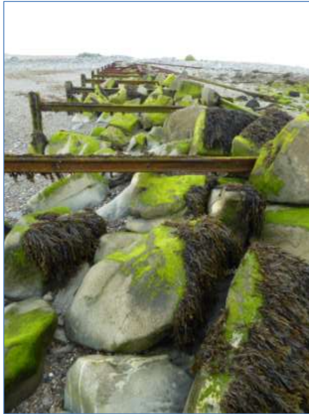
Plate 13: Armour rock within groyne structure
