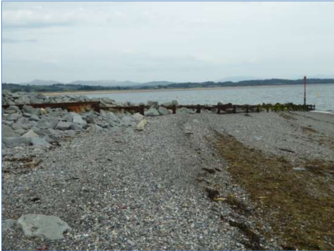
Plate 7: Side Elevation of Crib Groyne on Updrift Side
