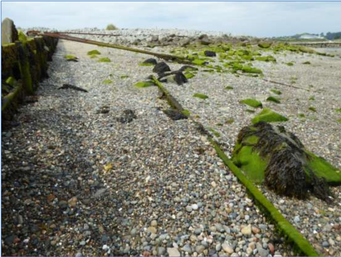
Plate 9: Foreshore on downdrift side of groyne, showing displaced walings and rock armour
