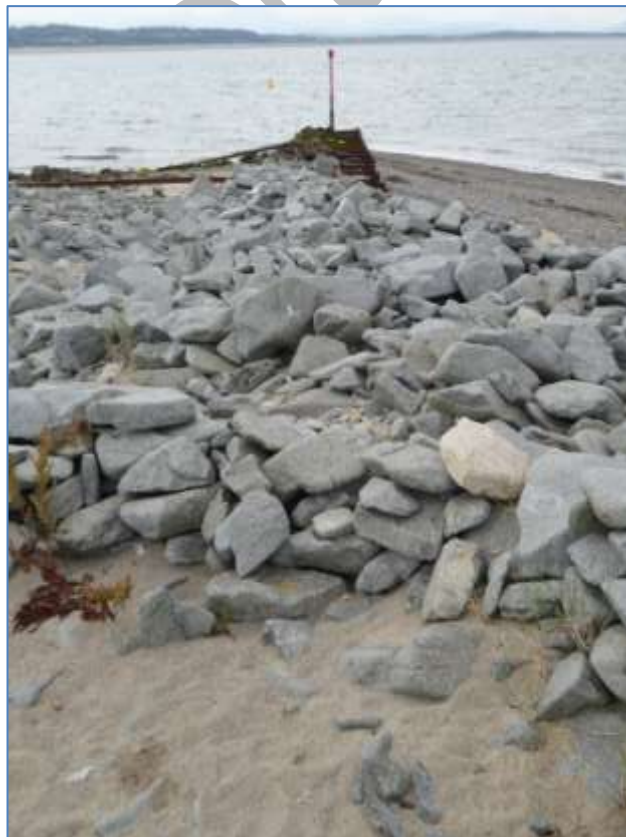
Plate 12: Rock protection mounded over landward section of crib groyne
