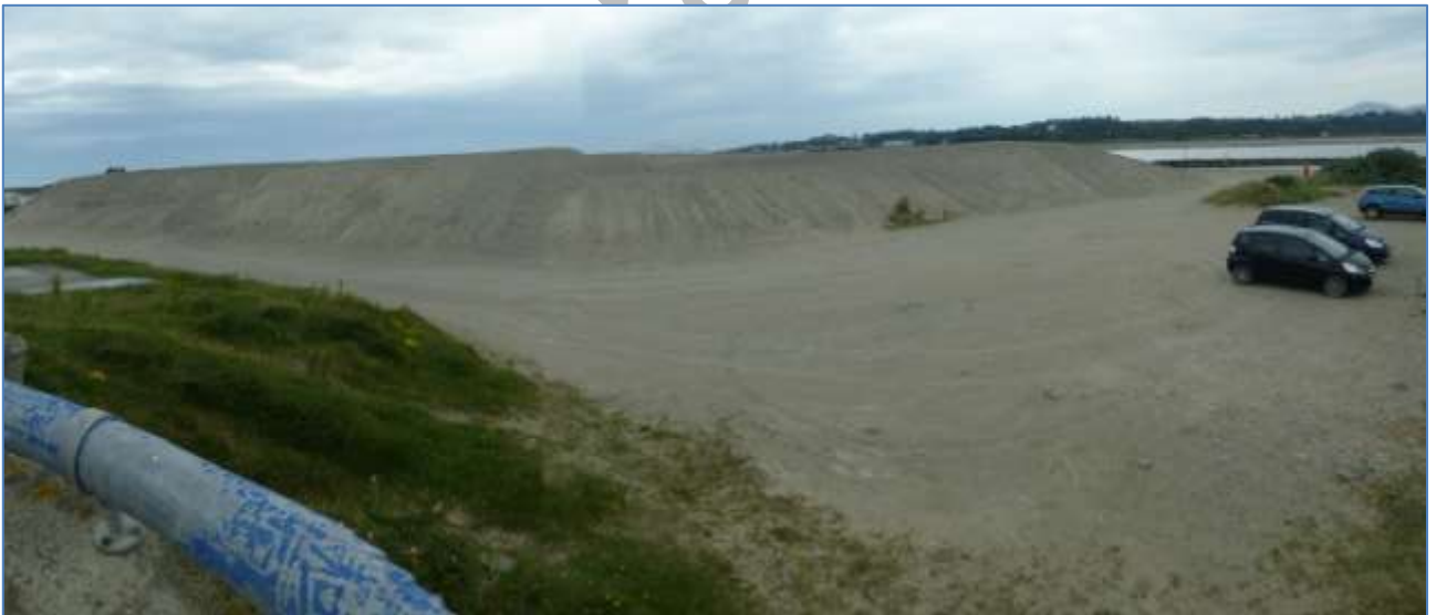
Plate 16: Stockpile of sand and shingle excavated from harbour mouth for recycling
